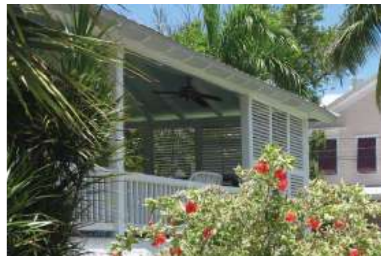
FIGURE 3.21 - Porch incorporates lowered enclosure walls to provide shade
