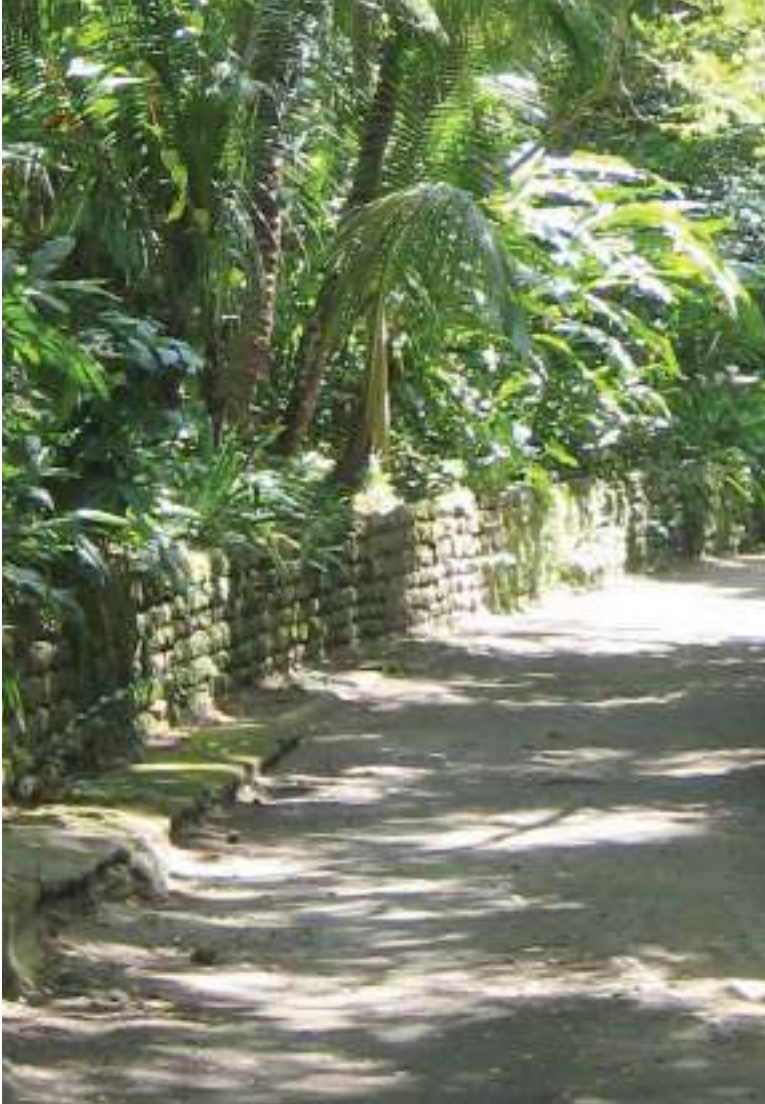
FIGURE 2.12 - Retaining wall utilizing regional stone
