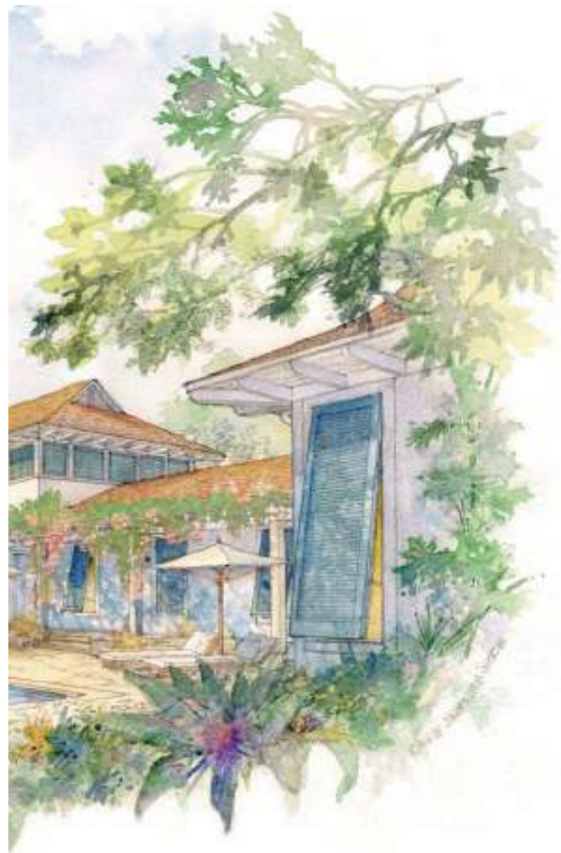
FIGURE 3.1☒ Awning provides shade while allowing for cooling breezes to enter
