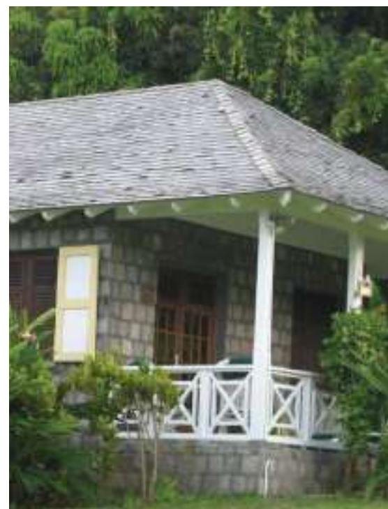
FIGURE 3.12 - Wood railing and posts combined with stone walls
