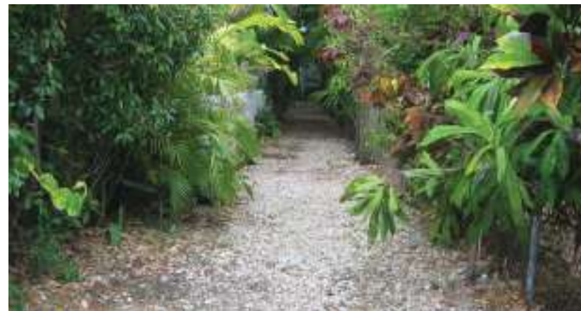
FIGURE 2.14 - Decomposed granite driveway
