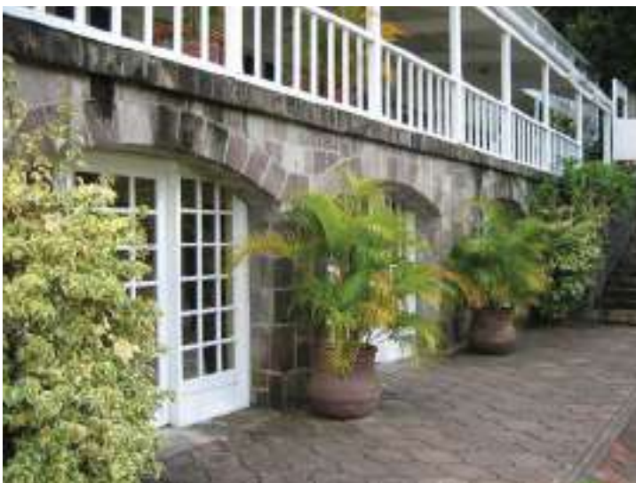
FIGURE 3.11 - Stone used on foundation level
